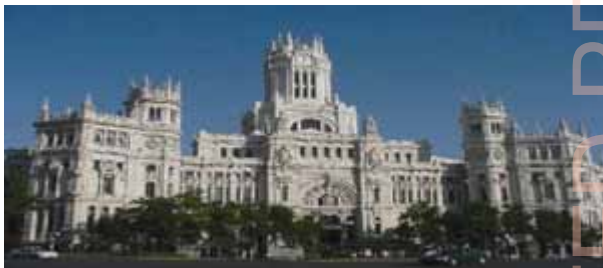
Figure 1: A general view of the building of study.
