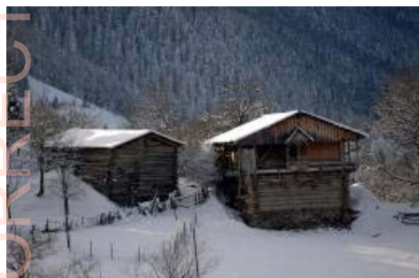
Figure 3. Some examples of rural houses in Artvin (Ozen, H.).
