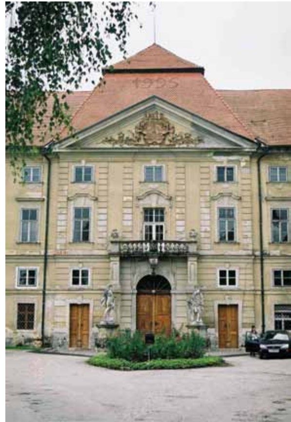
Figure 1: The view of the Novo Celje court from the north.
