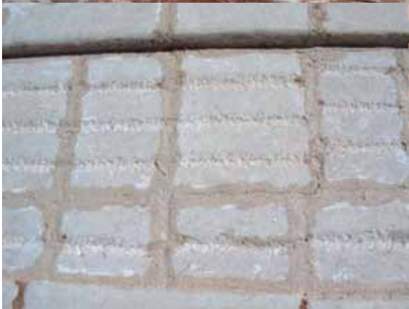
Figures 20-21: Construction of the pavement (above), with a detail (below).
