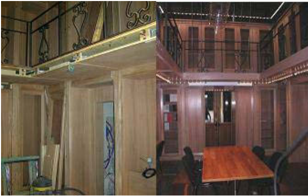
Figure 5: Conservation Hall. Indoor view during and after the works.
