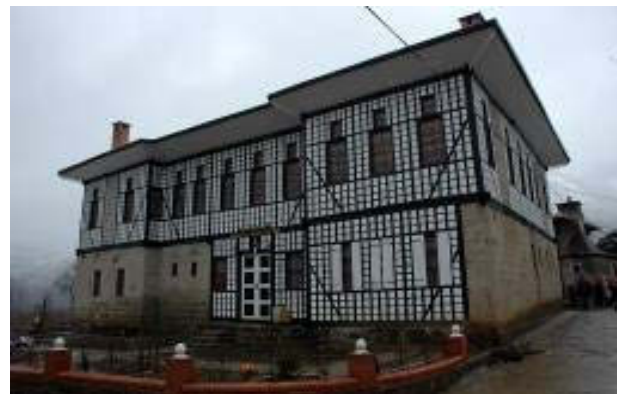
Figure 1: Some examples of rural houses in Trabzon (Ozen, H.).
