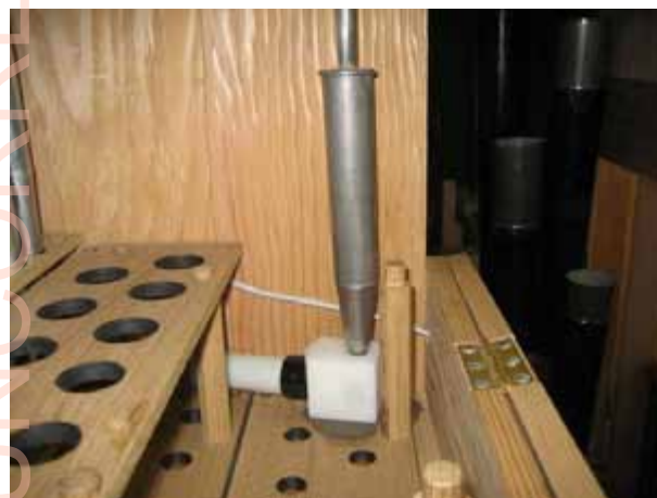
Figure 1: Location of holder in St Botolph without Aldgate. The empty holes represent places where pipes had to be removed and which had to be replaced after the installation. Within the PROPAIN "Improved Protection of Paintings during Exhibition, Storage and Transit" ( http://propaint.nilu.no ) project lead coupons and both lead and varnish coated crystals mounted in small holders (initially without continuous monitoring) were exposed in the microclimate frames. To test their response a model painting was prepared and freshly varnished and then placed in microclimate frames where air exchange measurements had been made. The lead coated crystals provided a response which was commensurate with the high
